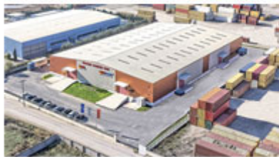
Warehouse in Thessaloniki - Greece
