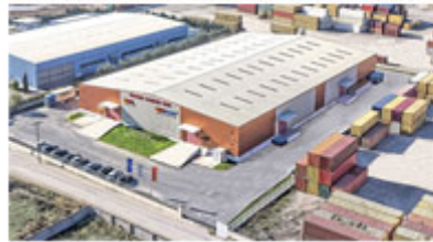
Warehouse in Thessaloniki - Greece
