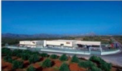
Central facilities – Factory in Chania – Crete- Greece
