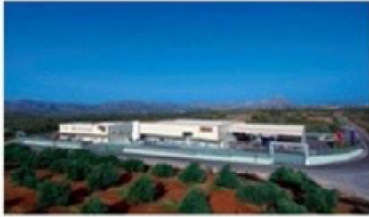
Central facilities – Factory in Chania – Crete- Greece
