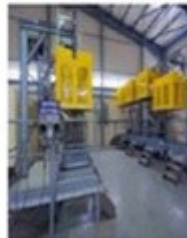
Gas Bottling Unit
