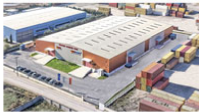
Warehouse in Thessaloniki - Greece
